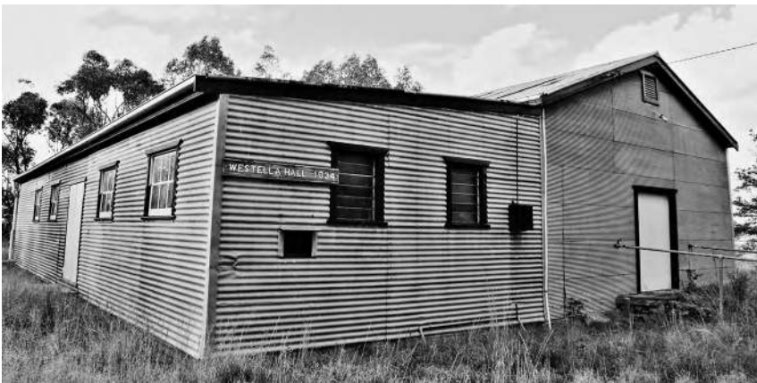
Figure 7.3: Westella Hall, with skillion extension of 1955.
