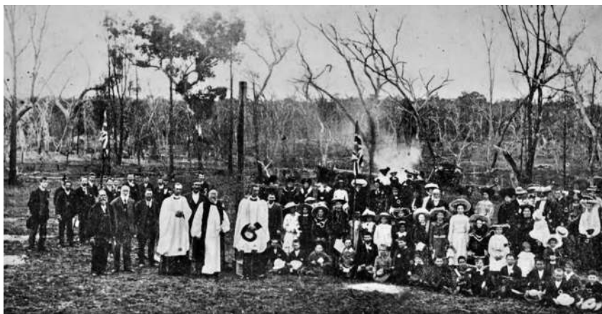
Figure 7.1: 'Laying of the corner post' of the Willandra Anglican Church, 1905.
