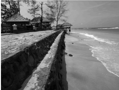
Figure 3.23 Site marked by left star in Figure 3.20, one year after installation. At start of the project, the seawall was being undermined and about to collapse. After one year, half a meter of sand had built up in front of it. Biorock Anti-Wave structures out of image, to the right. (Photograph by Tom Goreau, 2009.)
