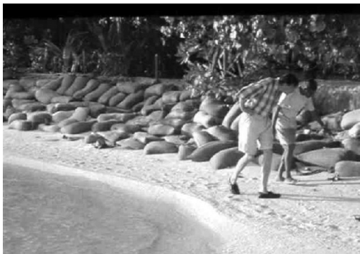
Figure 3.12 The beach on the south side of Ihuru Island before the start of the project in 1997. Sandbags have been piled in front of a meter and half high erosion scarp because trees were falling into the sea, and buildings about to collapse. (Photograph by Wolf Hilbertz.)
