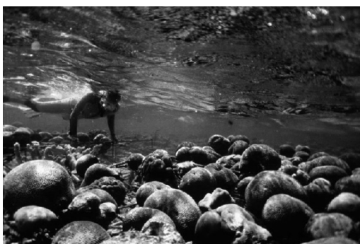
Figure 3.13 Necklace shore protection reef at Ihuru Island is located just in front of the eroding beach in the previous figure. Here, it is shown shortly after construction in 1997 after corals had been transplanted onto it. These corals were found loose on nearby reefs and attached to the Biorock structure. At this point, there is no limestone coating on the rebar. (Photograph by Wolf Hilbertz. For more photos of the development of this project see http://globalcoral.org/MALDIVES%20SHORELINES.%20GROWING%20A%20BEACH.htm .)
