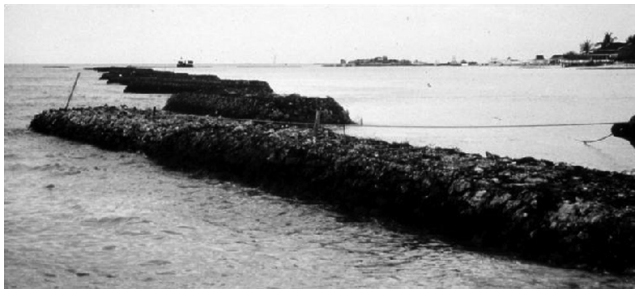
Figure 3.10 Breakwaters that surround Furanafushi Island, North Male Atoll, Maldives, now the Sheraton Full Moon Resort, are made up of corals mined from the reef. An entire reef was killed to make these walls. (Photograph by Wolf Hilbertz, 1997.)
