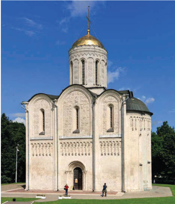
Figure 4: Cathedral of Saint Demetrios, Façade
