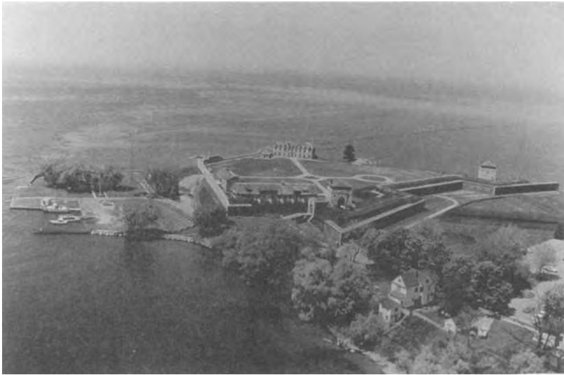
Aerial view of Fort Niagara, ca. 1990. OFN (dup) 7701/12. Courtesy Old Fort Niagara.
