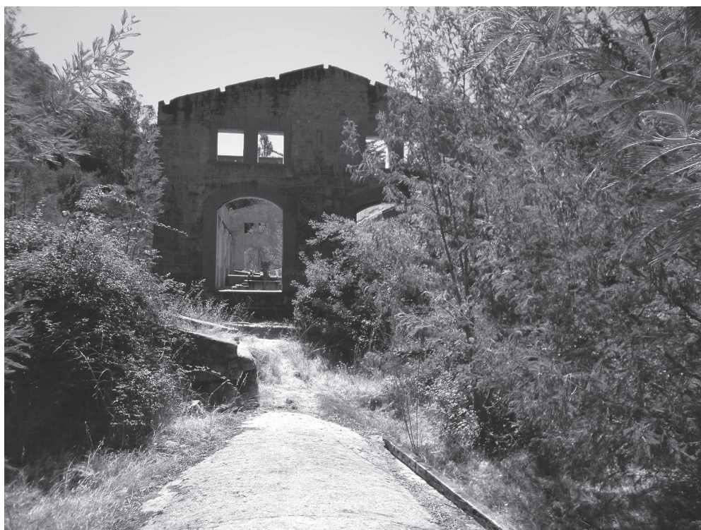
Figure 27.1 The machine hall of the El Sauce hydropower plant in the outskirts of Valparaíso, Chile. (Photo: author, 2014)
