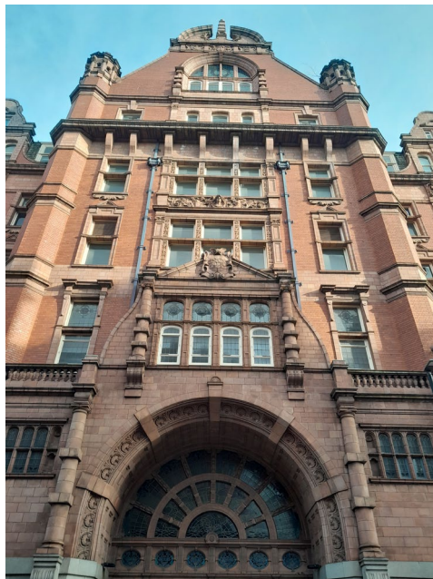
Fig. 5.28 Manchester Municipal Technical School, Sackville Street (Author, 2023).
