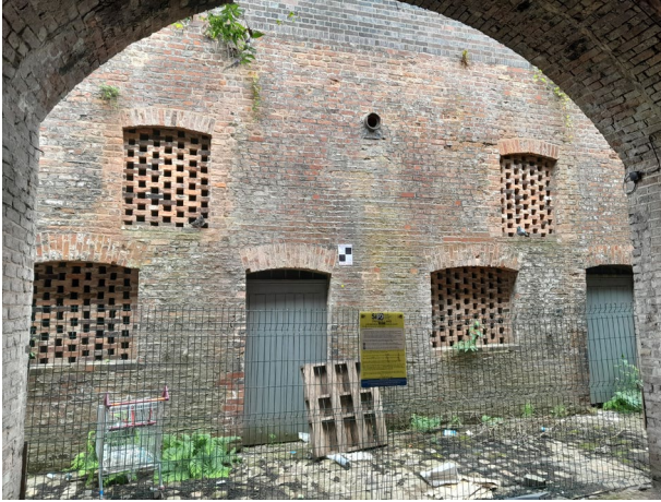
Fig. 2.52 Storerooms at the Arrivals Station, Water Street (Author, 2023).
