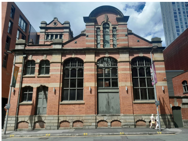
Fig. 5.24 Hydraulic Pumping Station, Water Street (Author, 2023).
