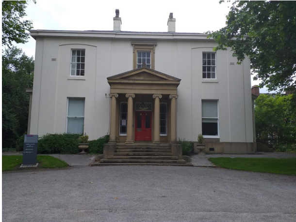
Fig. 2.47 Ashburne House, Fallowfield (Author, 2020).
