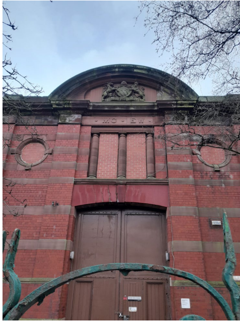
Fig. 5.26 Manchester Corporation Electricity Works sub-station, Heaton Moor (Author, 2023).
