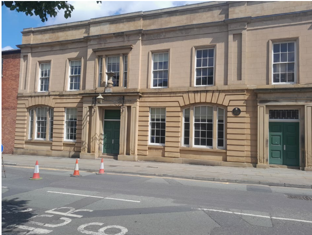
Fig. 2.50 Liverpool Road Station (showing the first- and second-class passenger entrances) (Author, 2023).
