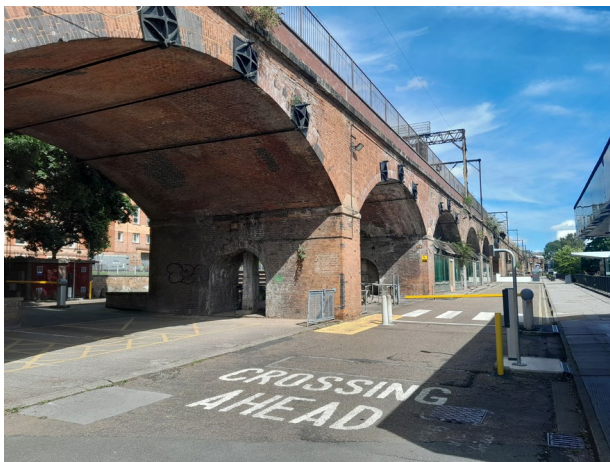
Fig. 3.9 Manchester South Junction and Altrincham Railway viaduct (Author, 2022).
