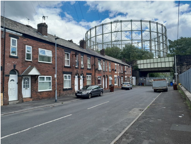
Fig. 5.22 Gas holder at Bradford Road Gas Works (Author, 2023).
