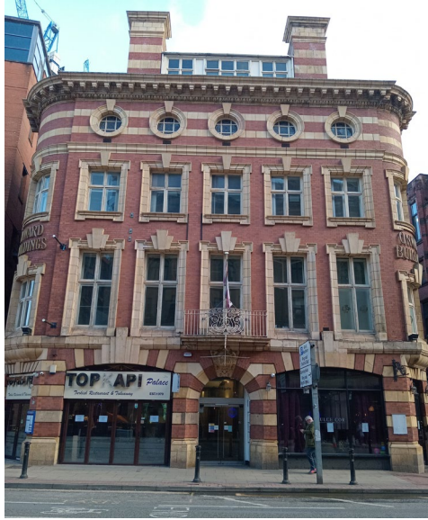
Fig. 5.53 Onwards Building, Deansgate (Author, 2025).
