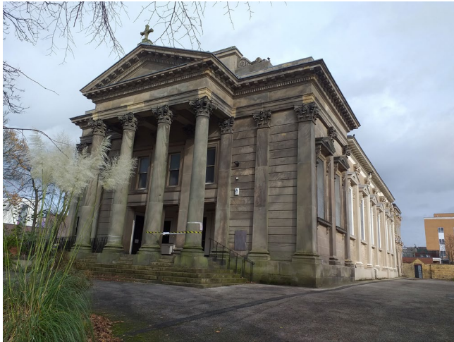
Fig. 4.48 Greek Orthodox Church, Bury New Road (Author, 2020).
