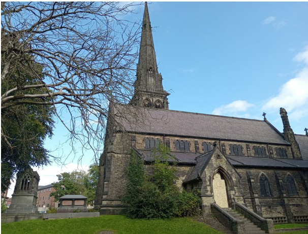
Fig. 4.20 Brookfield Unitarian Chapel, Gorton (showing the Peacock Mausoleum on the left) (Author, 2023).
