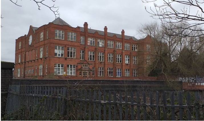
Fig. 4.33 Varna Street School, Openshaw (Author, 2021).
