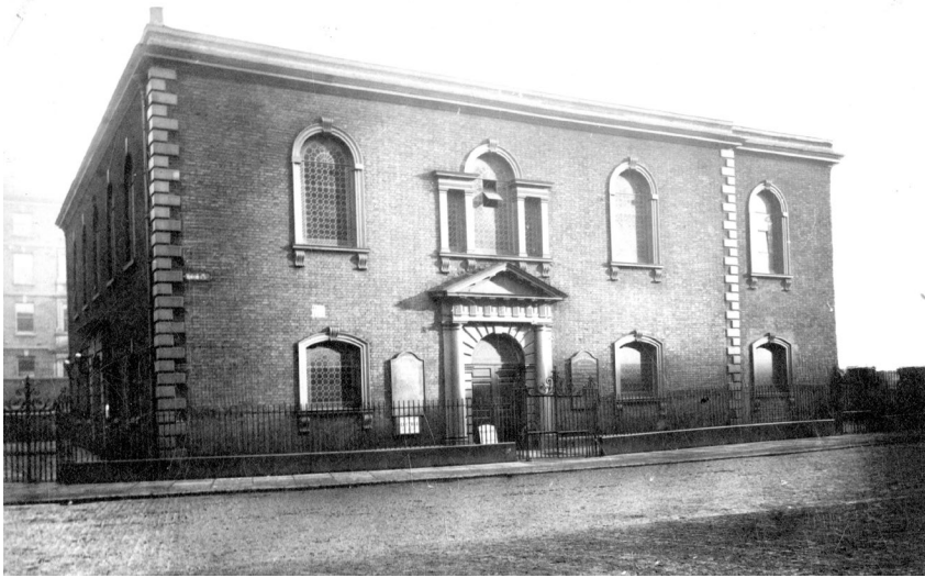
Fig. 1.7 Cross Street Chapel, 1900, unknown photographer. Image courtesy of Manchester Libraries.
