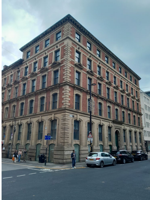
Fig. 3.11 12 Charlotte Street, palazzo-style warehouse (Author, 2022).
