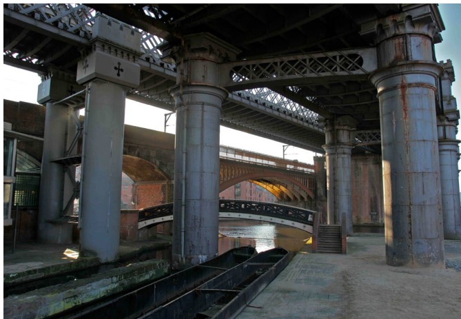
Fig. 5.9 Castlefield's railway viaducts (Author, 2011).
