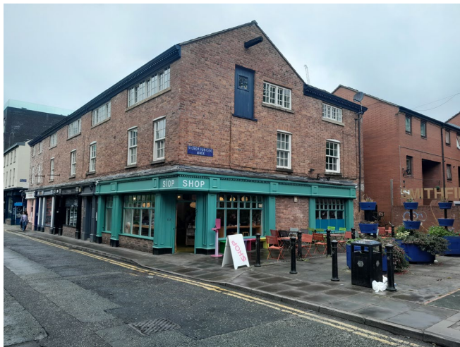
Fig. 2.8 47–53 Tib Street, Northern Quarter (showing workshop attic with windows and 'taking-in' door) (Author, 2022).
