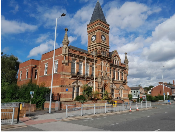
Fig. 4.30 Stretford Public Hall, Chester Road (Author, 2022).
