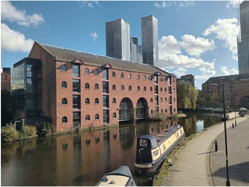
Fig. 2.12 Merchants' Warehouse (left) and the Middle Warehouse, Castlefield (Author, 2023).
