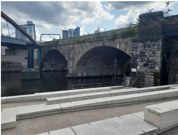
Fig. 2.51 River Irwell Railway Bridge (Author, 2023).
