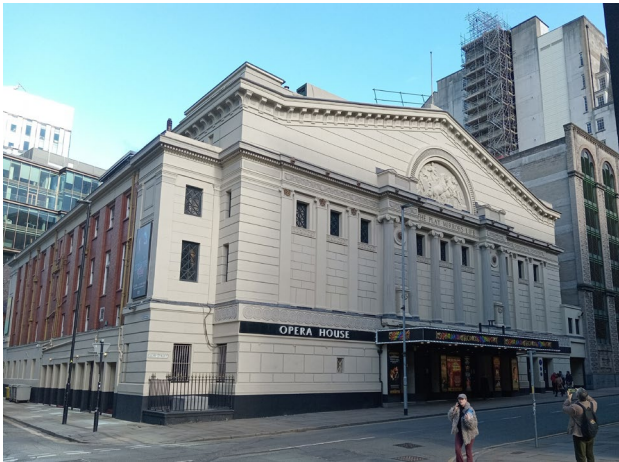
Fig. 5.39 New Theatre (Opera House), Quay Street (Author, 2025).
