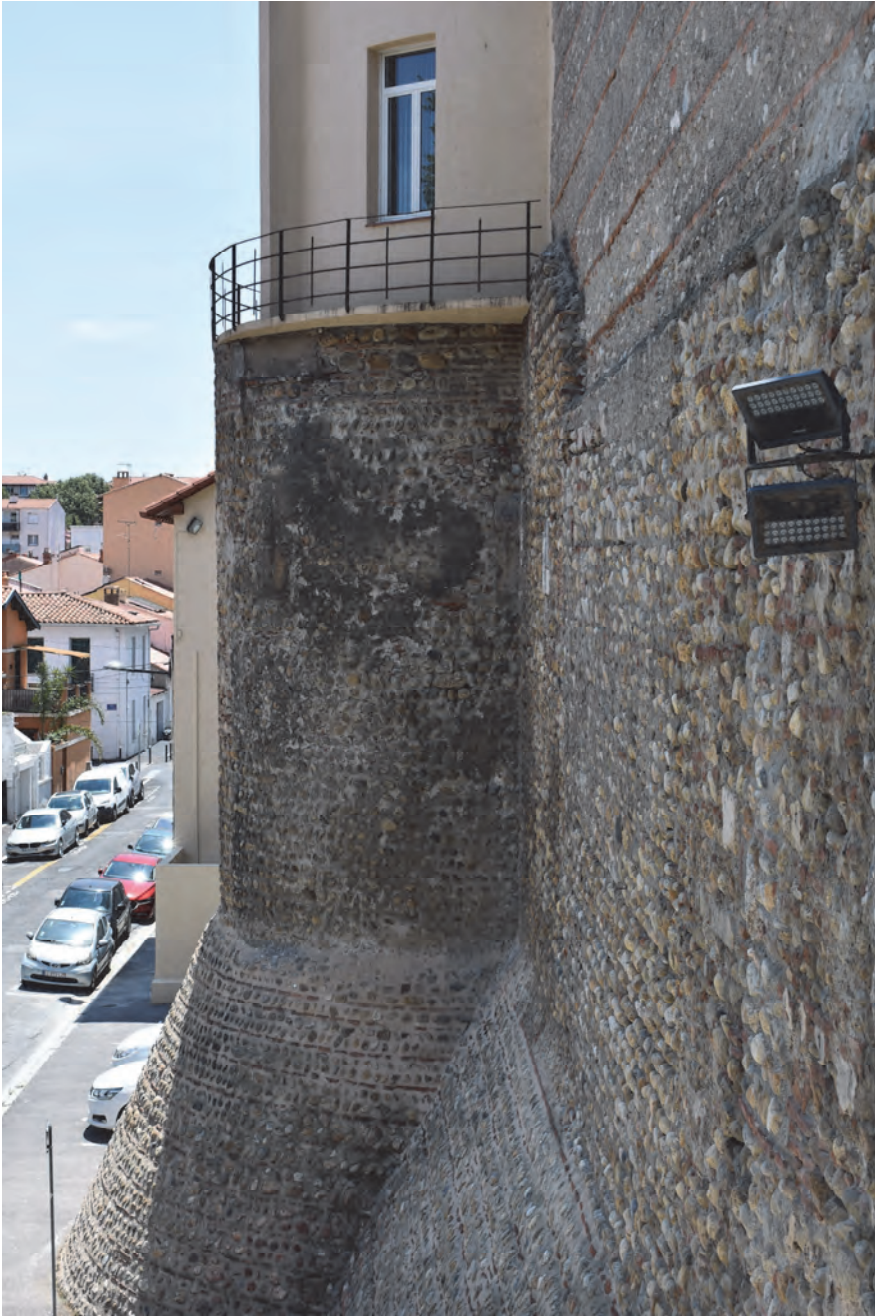
Fig. 10: Perpignan, remains of the northern city wall (photograph: author).
