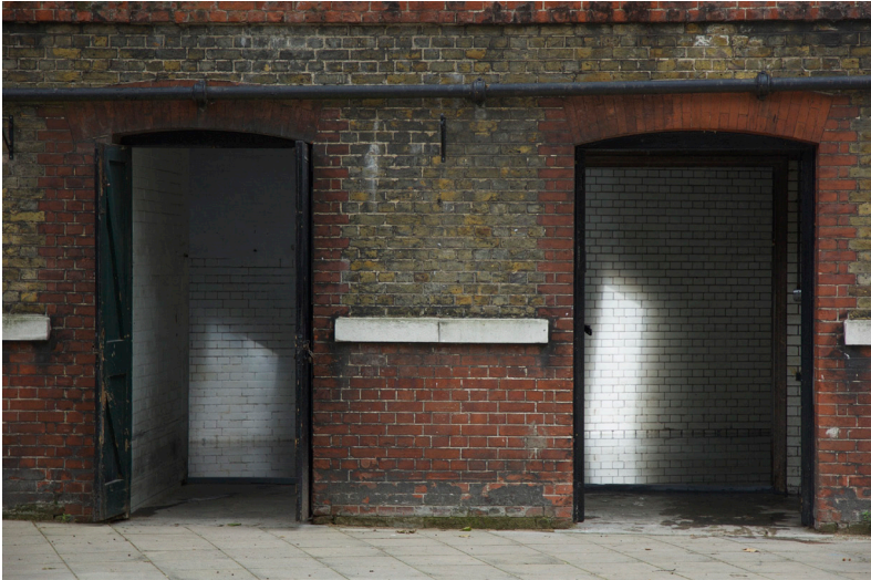
Figure 12.5 Ken Wilder, Skylights (2016). Exterior view of girls' and boys' mortuaries, Coram Campus, London. Source: © Ken Wilder.
