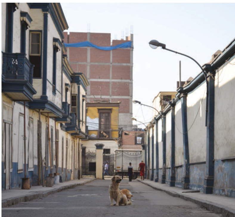
Figure 3.12 Emerging and often illegal storage facilities that deteriorate the residential character of Barrios Altos, Lima, 2020.
