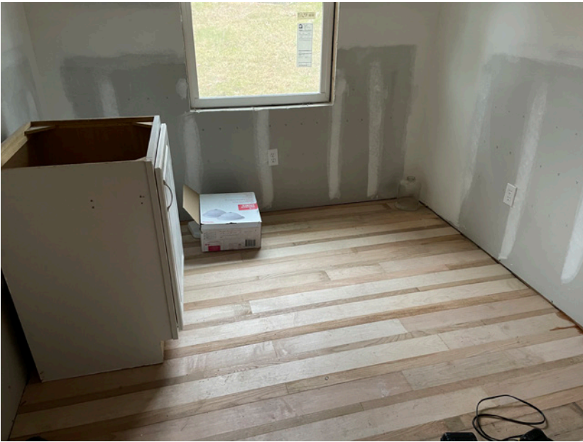
FIGURE 1.1. Photo of a mobile-home interior under renovation with hardwood floors and interior walls that are not made of engineered woods, December 2022. Photo by Nicholas Shapiro.
