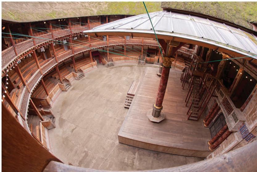
Fig. 8. The concentric circles of the new Globe. Visible at upper right is the lead pentice roof described earlier, which generated much debate among the design team over historical authenticity. Photo by Pete Le May. Courtesy of Shakespeare's Globe © 2018.
