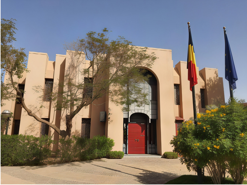
Figure 55: The Belgian embassy offices in Riyadh, 2022
