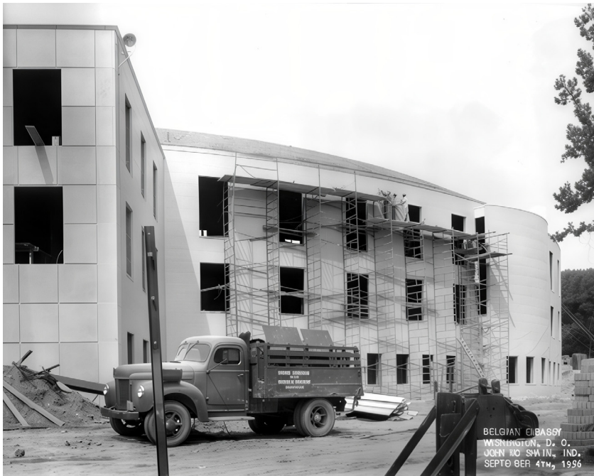
Figure 12: The chancery under construction, 4 September 1956
