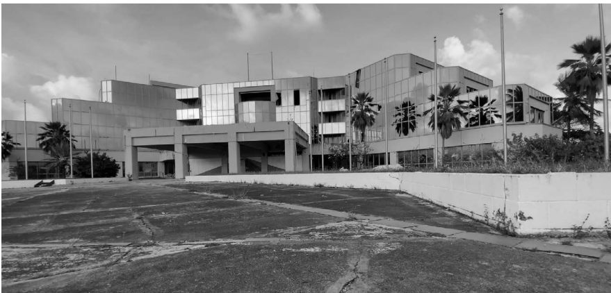
Figure 3.3 and 3.4 top: Kinked kerb and concrete platforms on the Northern flank of the capitol. Bottom: Ledges on the Southern flank of the plaza.
