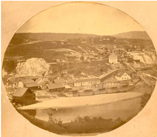
Figure 3.1: Photograph of the Blaafarveværket, Modum, Norway. In the centre of the picture are the calcination huts and arsenic refinery. To the left are the half-timbered colour mill, the stamping mill, the oxide hut and parts of the melting hut. From the centre, stretching across to the right, is a horizontal pipe called a poison catcher (photograph © Stiftelsen Modums Blaafarveværk; undated, but probably from the 1860s-1880s).
