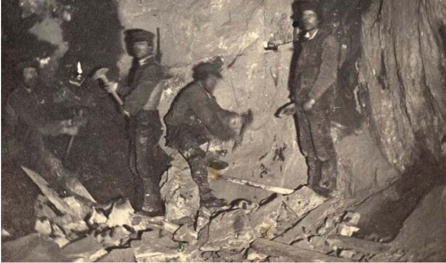
Figure 3.2: Photograph of four miners drilling by hand in the Blaafarveværket cobalt mines in Modum, Norway, in 1864. The men are dressed in woollen clothes and white shirts and are equipped with iron drills and sledgehammers. Their oil lamps hang on the mine wall next to them (photograph by Karl Gercke, 1864; © Stiftelsen Modums Blaafarveværk).
