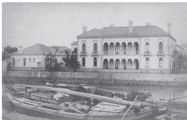
The Shibusawa house in Kabuto-chō (built in 1888). It was used as an office after Shibusawa moved to the family's new residence in Asukayama.
