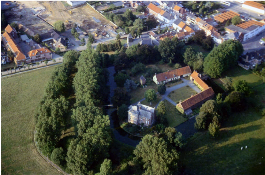
Figures 3, 4, and 5 Aerial photograph of the upper and lower courts of the seigneurie of Vichte (the original moat between the upper and lower courts has been filled in). The parish church lies to the north of the manor. Figure 4 shows the gatehouse. Figure 5 shows one of the great barns with the coats of arms of Jacob van Speelt and Florentina Wielant incorporated in the brickwork. (Philippe Despriet, V.Z.W. Archaeology South West Flanders; see also his publication De dorpsheerlijkheid , 22, 26–7).
