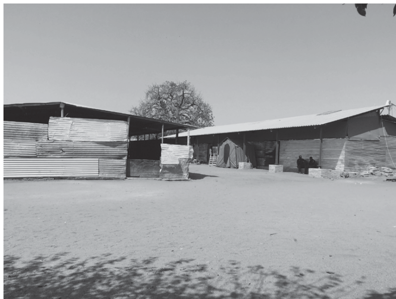
Figure 5.3: Outside image of the corrugated-iron shelter (right) next to the church (left) at the men's shelter
