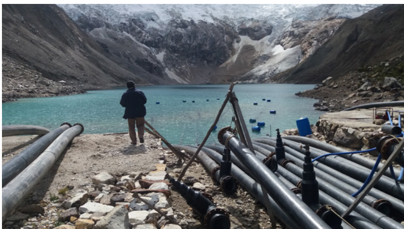
FIGURE 7.1. The siphons at Lake Palcacocha. (Photo by author)
