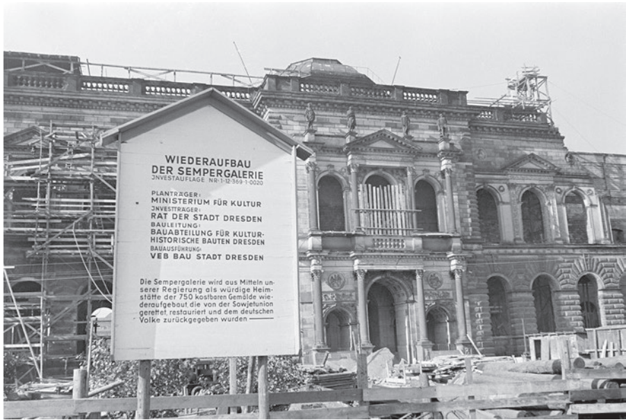
Fig. 26. Rebuilding of the Semper Galleries at the Zwinger (1956). (Photograph by Erich Höhne and Erich Pohl. Reprinted by permission of SLUB/Deutsche Fotothek.)
