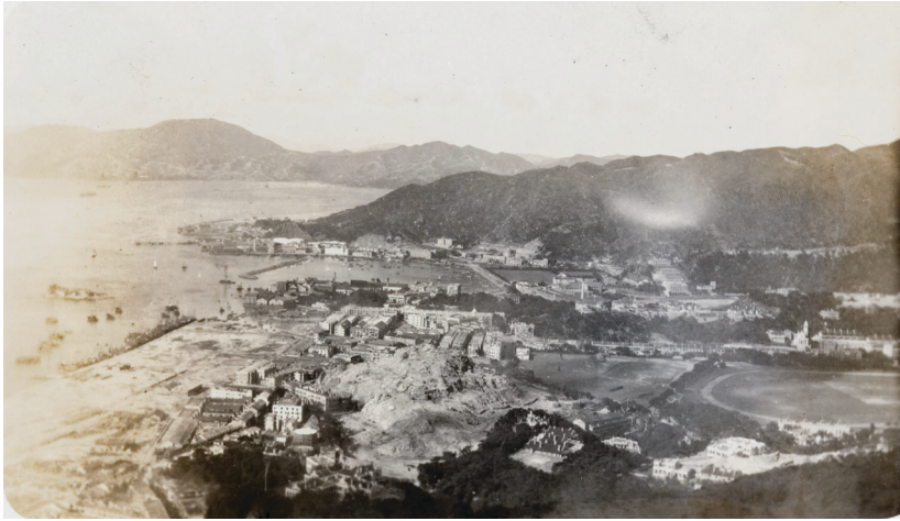
Figure 9.1: Land reclamation works, Hong Kong, 1933
