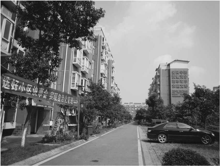
Compacted suburban communities for relocated farmers in a model site. Chengdu City, Sichuan.
