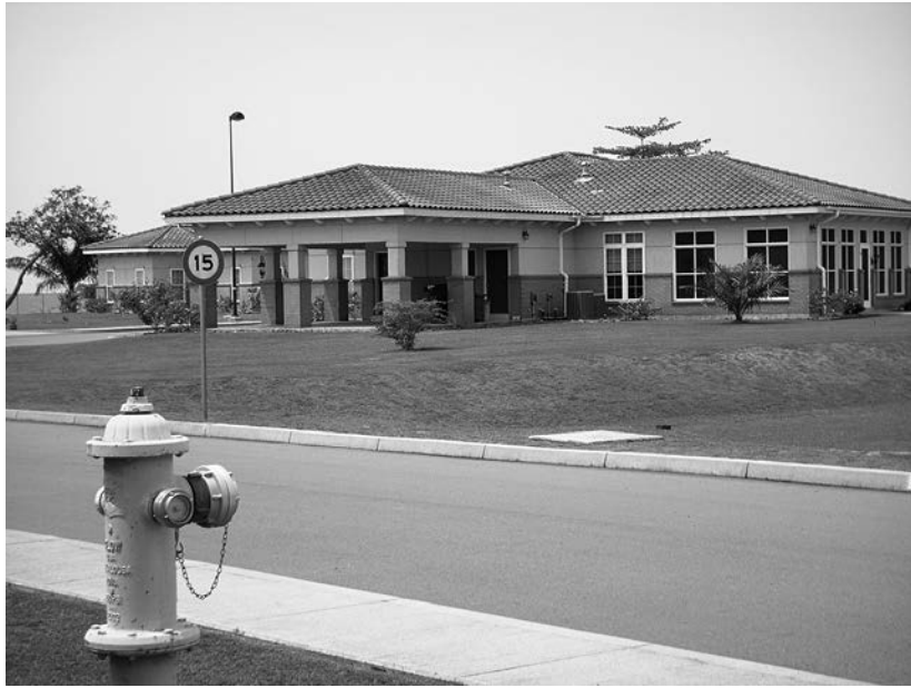
Figure 1.8. Fire hydrant and speed limit sign on the Smith compound.
