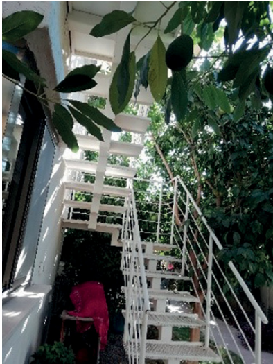
Figure 8.11 Illegal stairs in the backyard of a single-family (detached) home. Access to an illegally partitioned accessory housing unit, rented out. Location undisclosed. © Rachelle Alterman.
