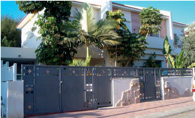
Figure 8.10 Next door – an example of an individually replaced fence, without a permit and noncompliant with the obligatory design. © Rachelle Alterman.
