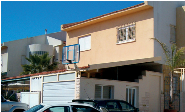
Figure 8.12 Garage illegally extended and converted into an accessory housing unit. Upper-middle-income neighbourhood in Netanya, Israel © Rachelle Alterman.
