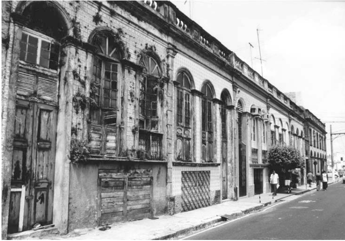
Fig. 4: Restored and dilapidated houses in the Cidade Velha (photo: Astrid Wonneberger)
