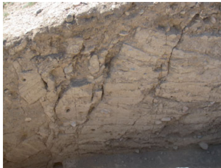
Fig. 7.6 Rammed earth wall of Tossor fortress (Lake Issyk Kul, Kyrgyzstan) as seen in excavation trench cross-cutting the buried wall. Layers are marked by horizontal scratches made by the excavating archaeologist. Three ruptures dissect the wall. Trench is 2.5 m deep (Photo M. Kázmér, #1246). For details see Korzhenkov et al. (2016)
