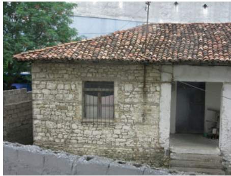
Fig. 7.10 Horizontal timber embedded in load-bearing wall masonry ( hatil construction). Wooden boards, when tied around the facade-side wall junctions aid in reducing the occurrence of corner wedge failures. These horizontal boards accept lateral loads during seismic shaking (Dogangün et al. 2006). Elbasan, Albania (Photo M. Kázmér, #8769)
