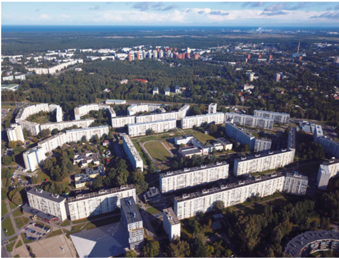
Fig. 8.3 Spatial organisation of mikrorayon Zolitūde II (arch. Berķe et al.) with school and kindergarten at the core. Source Sandra Treija
