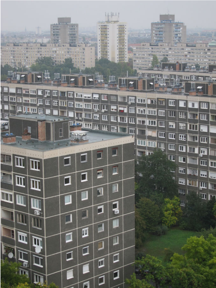
Fig. 6.2 Kelenföld, Budapest: pioneering prefabricated blocks built from 1965 using a Soviet spin-off of the Camus system Source M Glendinning, 2015
