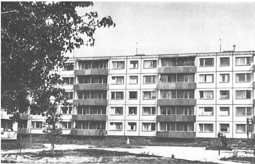
Fig. 4.4 An experimental large-panel apartment house (containing 75 units) based on standard series I-464. Source Žiburkus (1969), unpaginated
