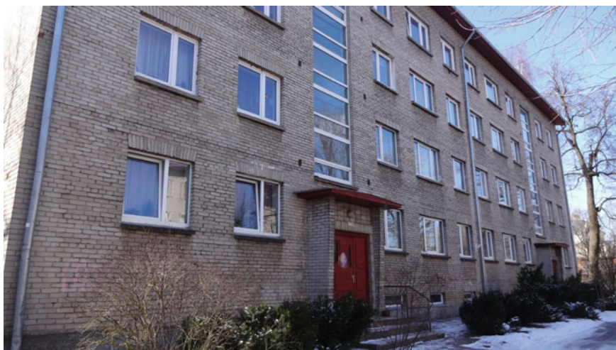
Fig. 17.1 A khrushchëvka apartment building in Tartu, Estonia prior to renovation (Tiigi 7, Tartu): a 4-storey, 32-unit building with 1,350 m 2 total floor space (an estimated 80 inhabitants live in the building). Source Photo by authors
