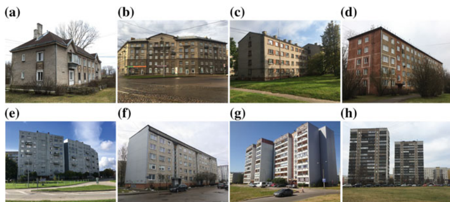
Fig. 11.3 Various types and series of Soviet-era apartment buildings in Riga. Note a typical two-storey apartment house built in the late 1940s; b solid stone building of the early 1950s in the Stalinist era, representing the architecture of Socialist Classicism; c typical apartment block of the Khrushchëv era in the late 1950s; d one of the first prefabricated-panel houses built in the early 1960s; e originally designated in Leningrad (Saint Petersburg); however, later, the apartment blocks of this series, the construction of which was widespread in the 1970s, became tied to Riga; f typical five-storey apartment block of the Brezhnev era in the 1970s; g nine-storey prefabricated-panel house of the 1980s; h the newest high-rise panel blocks of the late-Soviet period from the 1980s and early 1990s
