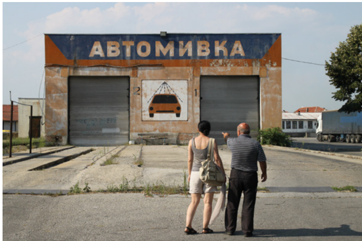
Fig. 18 Hieslmair and Zinganel, 2015 On tour visiting former SOMAT service stations all over Bulgaria: here in Pazardzhik in front of the former lorry wash station, with a doorman guiding the research team around the site which is partly abandoned today and partly used by other companies
