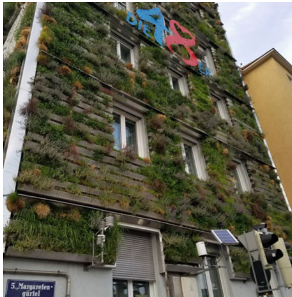
Fig. 1 “Climate façade” on the MA48 building, Vienna
