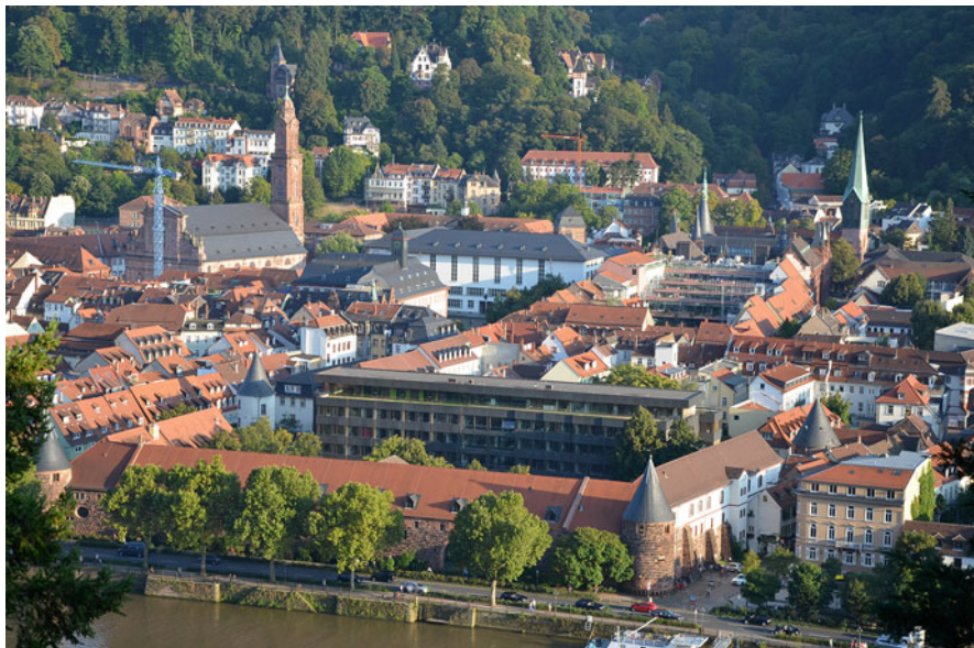
Fig. 14.2 Large administrative and faculty buildings of Heidelberg University, such as the Old University (1735), the New University (1931), and the Neues Kollegiengebäude (1965), alter the urban fabric of the Old Town. Debate continues about the direction in which the next leap forward is to go (e.g., the urbanization of monofunctional campuses?). Source and copyright: Carl Zillich.
