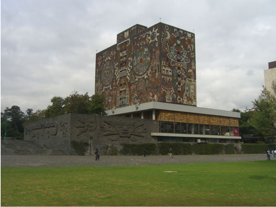
Fig. 12.50 Central library of the National Autonomous University of Mexico on the Mexico City campus (built by Juan O’Gorman).
