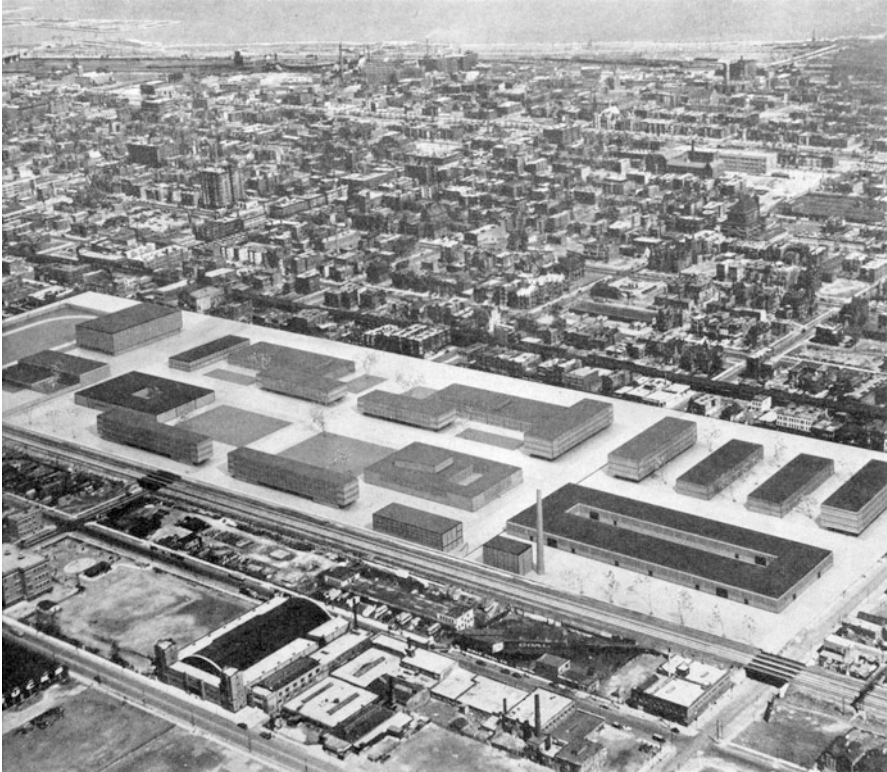
Fig. 12.48 Mies van der Rohe, Project for the Illinois Institute of Technology campus in Chicago. Final scheme, 1940.
