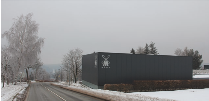
Picture 1 MÜHLE premises in Hundshübel (picture by author)
