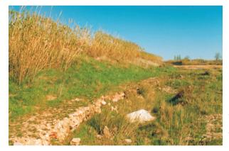
Photo 3.7 – River Agly dike inspection following flooding on 12-13 November 1999: exposed foundation anchor block made of rip rap, at the foot of a bank.
