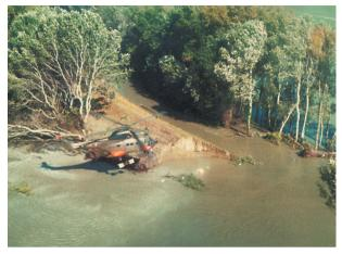
Photo 2.11 (Source: Service Navigation Rhône-Saône) – Internal erosion (animal burrows or warrens, conduit crossings) was found to have caused all 16 breaches in the Camargue dikes during the two Rhône floods in the winter of 1993-1994.
