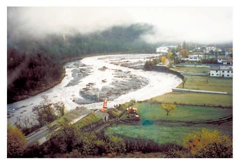
Photo 2.6 (Source: ONF Alpes Maritimes) – Eroded bend caused by flooding of the River Var on 5 November 1994: the Guillaumes dike (Alpes Maritimes) with over 150 metres of the D2202 roadway swept away.
