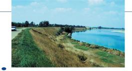
DIKE: An artificial structure, flood protection embankment or barrier that protects against river flooding, at least a part of which is built above natural ground level. It is designed to periodically contain a high discharge of water and thus protect areas that are naturally prone to flooding. (The term "levee" is often used along the French River Loire in common with certain areas of the USA).
