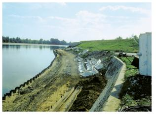
Photo 6.10 – Protection in the process of construction at the base of the river-side slope of the Val de Bou levee.
