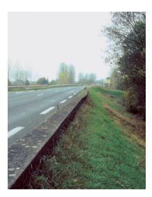
Photo 3.19 – Unstable freeboard masonry wall on the Authion valley levee (Maine-et-Loire)
