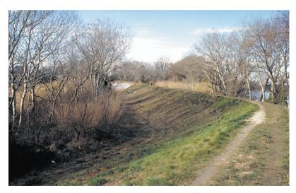
Photo 1.2 – Fill dike on the Petit Rhône in the Camargue (Bouches-du-Rhône), prior to upgrading work in 1994. Its crest is too narrow to allow plant and machinery to pass.
