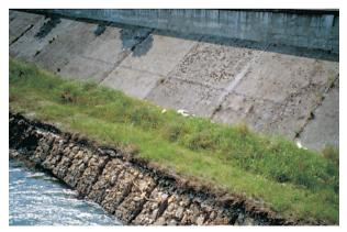
Photo 3.8 – Scouring at the foot of a protected bank on the Gardon d'Alès – gabion protection in poor condition.
