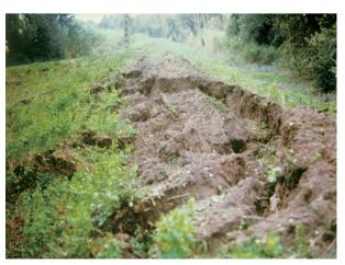
Photo 2.16 (Source: DDE 13) - Embankment landslide affecting the crest of the structure (Camargue dike).
