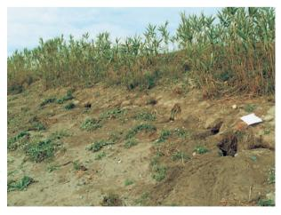
Photo 5.5 – Animal burrows can cause serious damage if numerous and/or large and in places where embankments are narrow in section.
