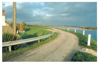
Photo 3.15 - Section of the Val de Bou levee on the right bank of the River Loire, made narrower because of the presence of a house on the land side: a potentially vulnerable spot to be inspected during flooding.
