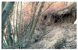
Photo 3.16 - Escarpment and leaning trees on a river bank or on the river-side slope of a dike indicate general slope instability following the retreat of flood waters.
