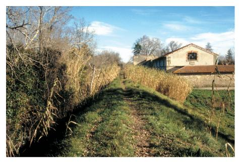
Photo 5.1 – Dense ground cover (in this case, giant reeds) makes it very difficult to visually inspect this dike on the Petit-Rhône.
