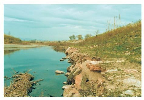
Photo 2.7 – River Agly dikes: foundation anchor block made of rip-rap at the foot of a bank partially swept away during flooding on 12-13 November 1999.
