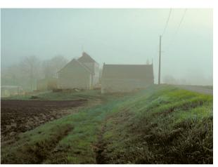
Photo 1.9 – Construction embedded in the land-side slope of a River Cher levee at Savonnières (Indreet-Loire).
