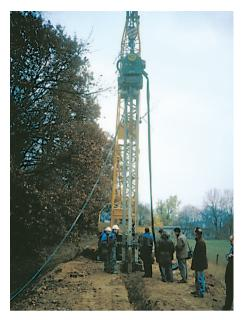
Photo 6.12 – Construction of a narrow diaphragm wall to create a seal in the body of a dike (Oder levee, Poland).
