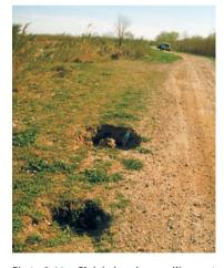
Photo 3.11 – Sink holes along a dike crest are often a sign of internal erosion. Here, two sink holes appeared in the Agly dike crest within a few weeks of each other after the flood of 12-13 November 1999.
