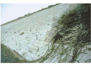
Photo 6.14 – River-side stone facing repaired with pre-fabricated elements on the Authion Valley levee.
