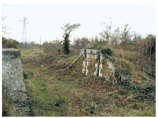
Photo 1.11 – Closable track on the right-bank dike of the Grand Rhône at Salins-de-Giraud (Bouches-du-Rhône).
