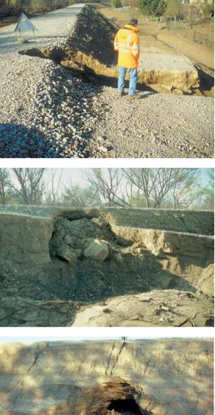
Photo 2.8 (Cemagref: Cyril Folton) – Damage caused by tunnel erosion (piping) in the new dike at Cuxacd'Aude during flooding on 12-13 November 1999. A badly-installed conduit crossing was found to be the cause.
