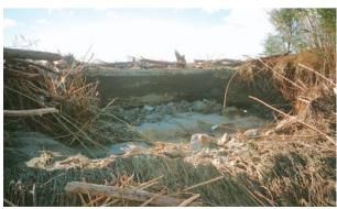
Photo 3.1b (Source: DDE 66) – Detail of the eroded zone shown in the previous photo, revealing layers in the dike composition.
