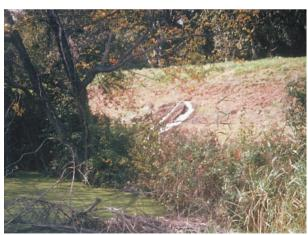
Photo 2.13 (Source: Service Navigation Rhône-Saône) – Leak on the downstream face of a Camargue dike caused by animal burrowing.
