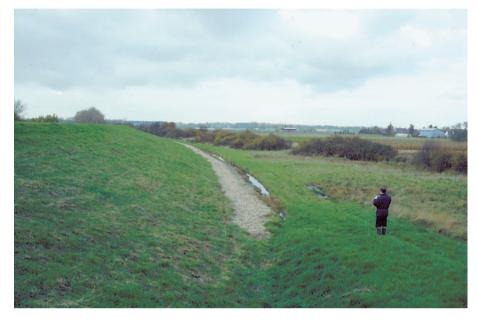
Photo 6.7 - Widening of the land-side slope over a drainage blanket - Val de Bou levee.
