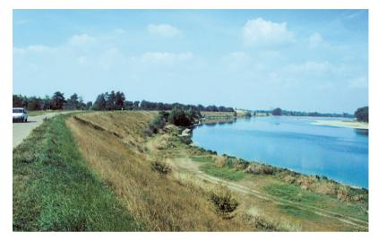
Photo 1.1 – Typical view of a levee on the middle reaches of the Loire: fill dike with a broad cross-section, grassed slopes and crest roadway.
