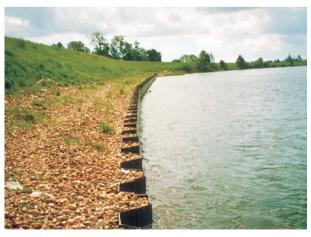
Photo 6.11 – Sheet piling as a protection for the base of the left-bank levee in St-Benoît (Loiret).
