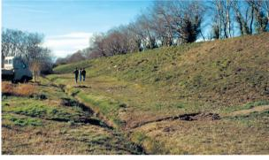
Photo 3.10 – Inspection of the Petit Rhône dike near Arles after flooding on 8 January 1994: evidence of seepage across the embankment at the toe of the land-side slope.
