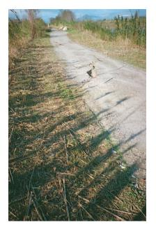
Photo 3.18 – Crack formation on the crest of a dike following the retreat of River Agly flood waters in November 1999 – sign of river-side slope instability following a rapid fall in the river water level.
