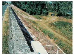
Photo 2.17 (Cemagref, Rémy Tourment) – Freeboard masonry wall on the river-side crest edge of the Val de Cisse levee (Indreet-Loire). Access to the river in the background.
