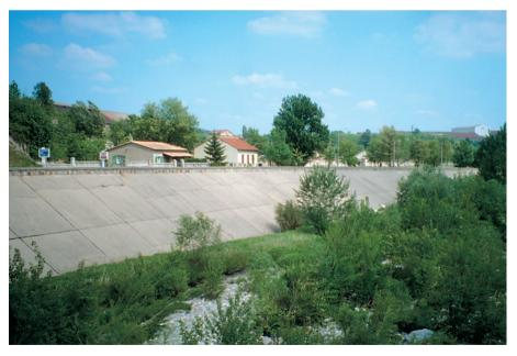
Photo 1.6 – Work dating from 1958 on the Gardon river as it passes through the town of Alès (Gard): the bank is protected by concrete slabs that only locally serve as a dike.
