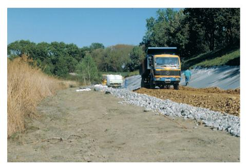
Photo 6.8 – Emergency construction of a downstream drainage shoulder at the toe of the land-side slope of the Petit Rhône dike following the flood of 8 January 1994.
