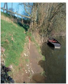
Photo 3.6 – When old stone facing is exposed at the base of a river-side flood embankment, it may indicate undermining by the watercourse.
