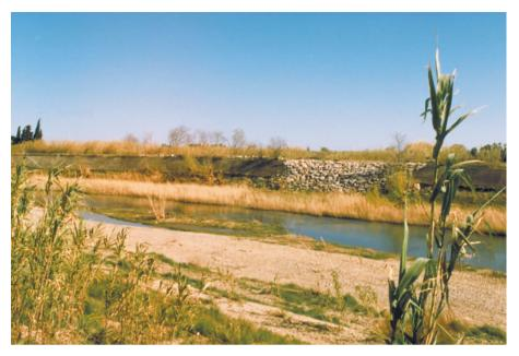
Photo 1.5 – Old concrete protection on the bank and river-side slope of the Agly right-bank dike (Pyrénées Orientales). Recent repairs have been made in riprap.
