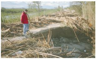
Photo 3.1a (Source: DDE 66) – Damage caused by overtopping on the River Agly dikes following flooding on 12-13 November 1999. Extensive eroded zone in the embankment and high-water debris left on the crest.
