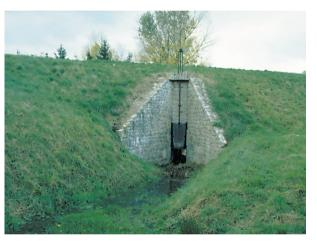
Photo 1.10 – Closable sluice in a Loire levee at Val de Bou (Loiret), seen from the land side.
