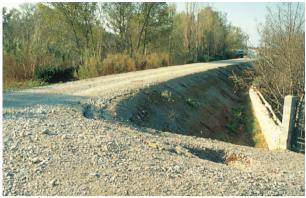
Photo 3.9 – Sink hole and collapsed areas on the land-side top of the dike at Cuxac d'Aude after flooding on 12-13 November 1999. A conduit crossing was the cause of the damage.
