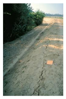
Photo 3.17 – Slopes with a gradient that is too steep (river side in this case) expose the dike to the risk of instability.
