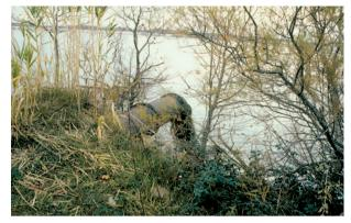
Photo 3.13 - The passage of pipes through embankments (here, a Photo 3.14 - A non-return valve pumping station conduit drawing water from the Grand-Rhône) are outlet at the toe of the river-side points to be given particular attention during inspections.
