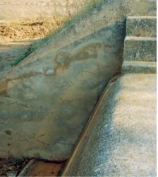
Photo 3.4 – Spillways need to be carefully inspected after flooding. Here, muddy traces left on the side wall make it possible to estimate the peak spillover height.
