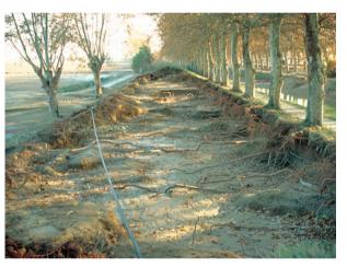
Photo 5.4 – The breaches at Sallèles-d'Aude revealed the roots of plane trees running right the way through the base of the embankment.
