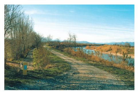
Photo 5.2 – Service tracks along dike crests (and in this case along the land-side toe of the embankment) facilitate surveillance operations on the River Agly.
