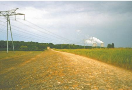
Photo 1.7 – Masonry spillway at Ouzouer-sur-Loire (Loiret), with erodible earth ridge (grassed bank on the right of the photo) called "banquette" in France.
