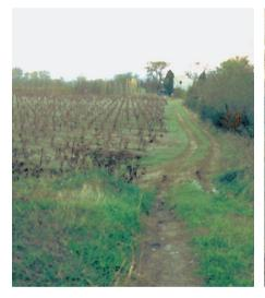
Photo 3.3 – Post-flood inspection of the Cuxacd'Aude dike: low points on the crest (passage of pathway) where overtopping occurred.
