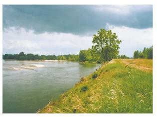
Photo 2.4 – Toe of a dike in contact with the main channel of the Loire on a concave bend of the Espagne levee at La Charitésur-Loire (Nièvre).
