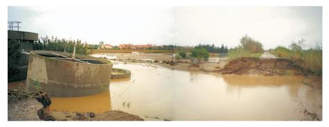
Photo 2.2 – Panoramic view (courtesy of Éric JOSSE, DDE 66) – Cross-section of the breach caused by overtopping at St-Laurent-de-la-Salanque on the left-bank dike of the Agly and damage to the waste-water treatment plant.
