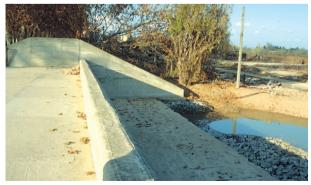
Photo 3.5 – Spillway at Sallèles d'Aude after flooding on 12-13 November 1999, showing damage to the gabion-built protective invert.
