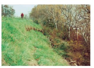
Photo 2.15 (Source: DDE 13) – Landslide following the retreat of flood waters – river-side slope of the left-bank dike of the Grand Rhône at Mas de la Ville.
