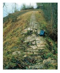
Photo 3.12 – Collapsed area on a masonry crest on a River Allier dike at Moulins (Allier), indicating internal erosion and/or settling of earthfill materials.
