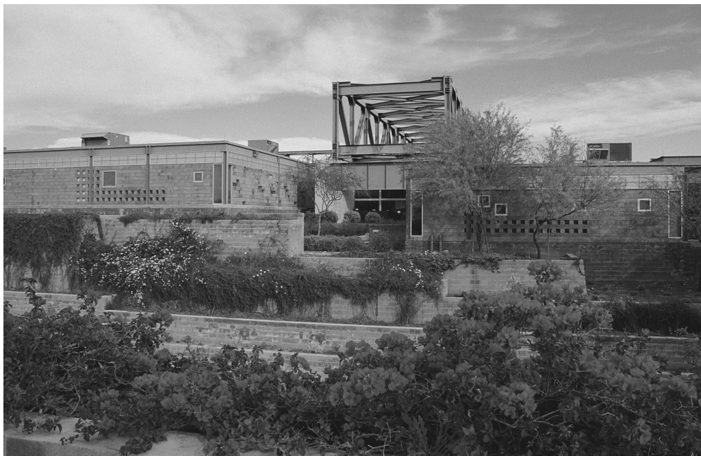
3.11 Solid Waste Transfer and Recycling Center, Phoenix, Arizona Michael Singer with Linnea Glatt, 1989–1993
