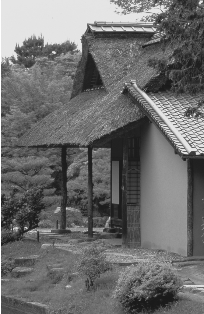
1.10 Shokin-tei, Katsura Villa, Kyoto, Japan, seventeenth century. The stepping stones direct movement from the boat landing into the tea house
