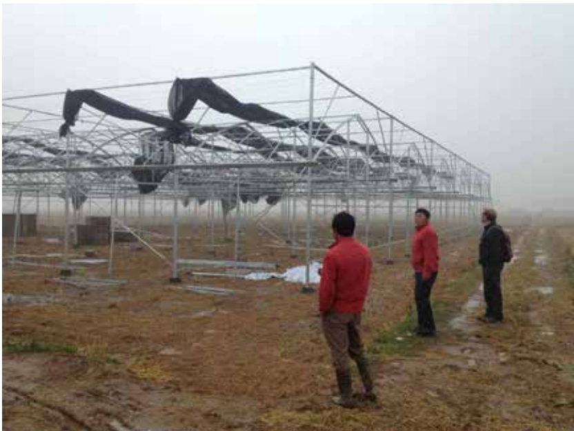
Figure 3.2 Construction of a large modern vegetable greenhouse in the AT
