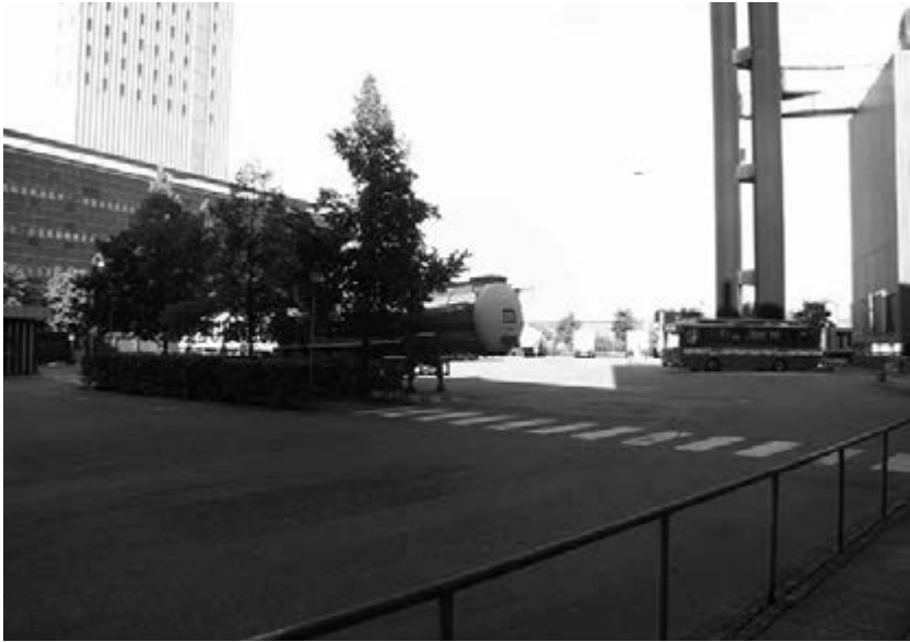
Figure 16.3 Two Chimneys Evaluated
