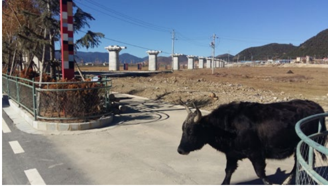
Railway under construction with yak in foreground Photo: Ben Hillman
