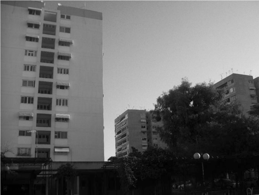
Fig. 4.4 Ten-storey condominiums in Tavros built between 1969 and 1971 by the Ministry of Social Care, 2016. Source Myofa, personal archive, 2016
