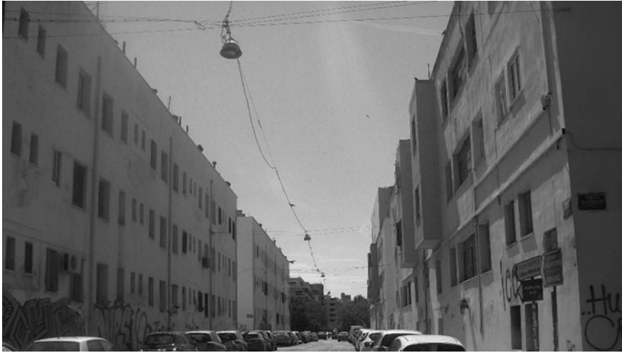
Fig. 4.1 The first four condominiums in Dourgouti, part of the old public housing stock for refugees constructed between 1935 and 1936 by the Ministry of Social Care, 2016. Source Myofa, personal archive, 2016
