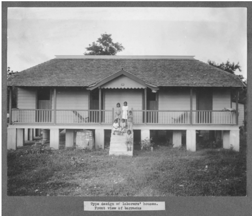
Figure 1: Type design of labourers' houses. Front view of barracks.
