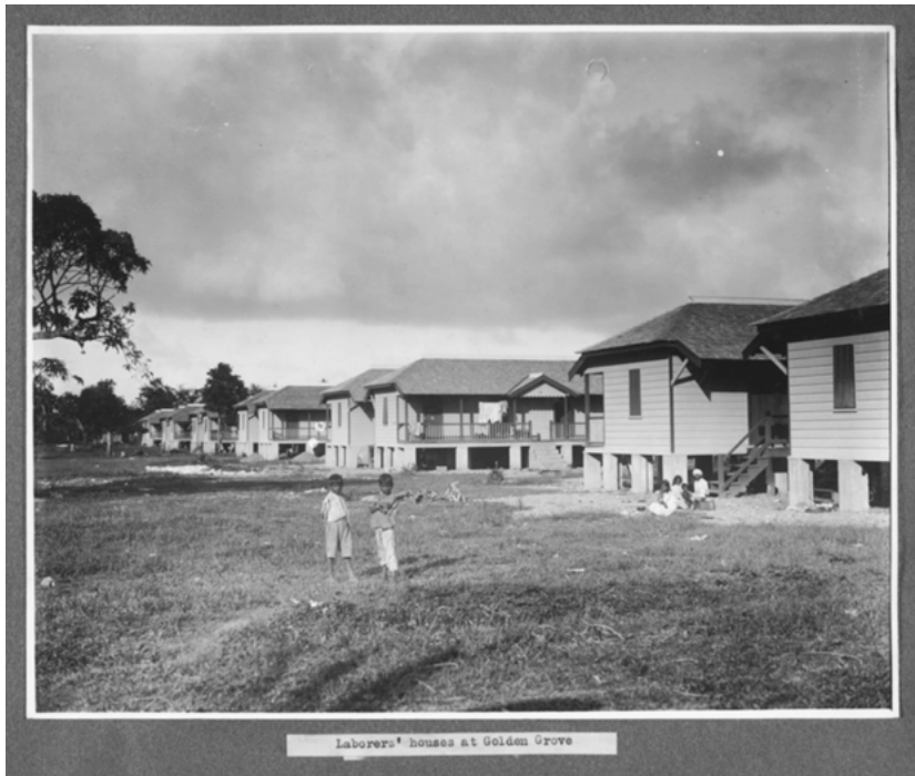
Figure 2: Labourers’ houses at Golden Grove
