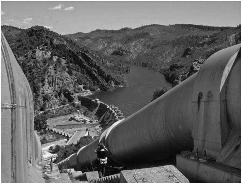
Figure 4.3 Bolarque Dam in the Tagus River and intake point for the Tagus-Segura aqueduct. Source: Author Leandro Del Moral.
