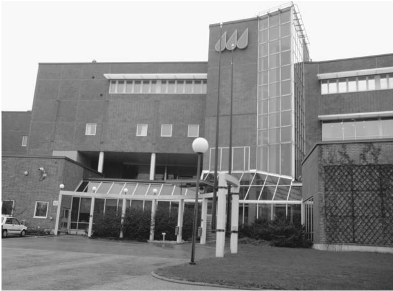
Figure 16.3 Head office of Viikinmäki Waste Water Treatment Plant in Helsinki. Source: Photograph Rajala, 2007.
