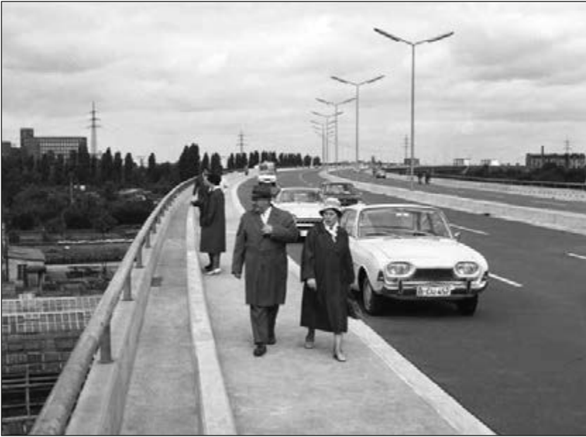
3. Bauwochen exhibition tour of the urban motorway between the Funkturm and Jakob-Kaiser-Platz, at the 'Nordwestbogen' bridge in Charlottenburg. 9 September 1962. Photograph: Karl-Heinz Schubert. Courtesy of Berlin Landesarchiv.
