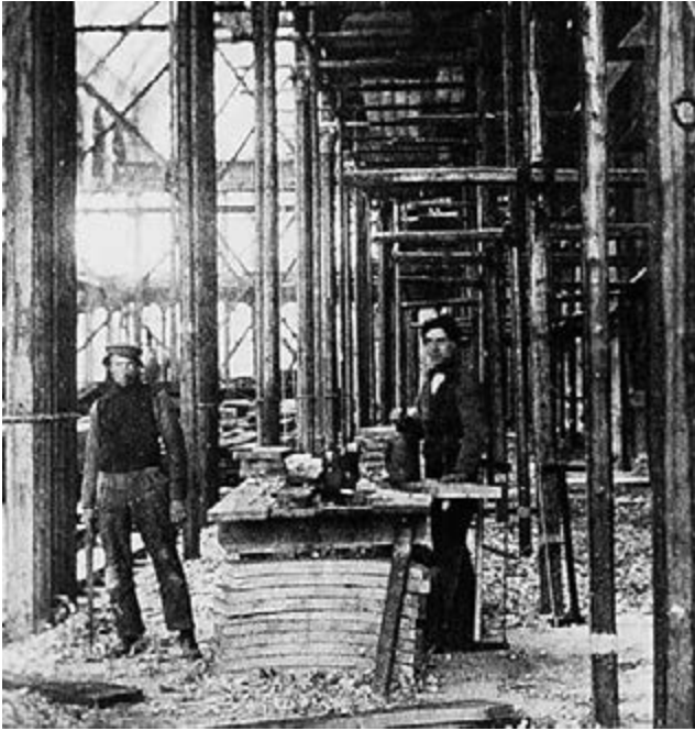
Figure 3.1 Carpenters at the construction of the Paleis voor Volksvlijt (Palace of People's Industry), Amsterdam, c. 1862
