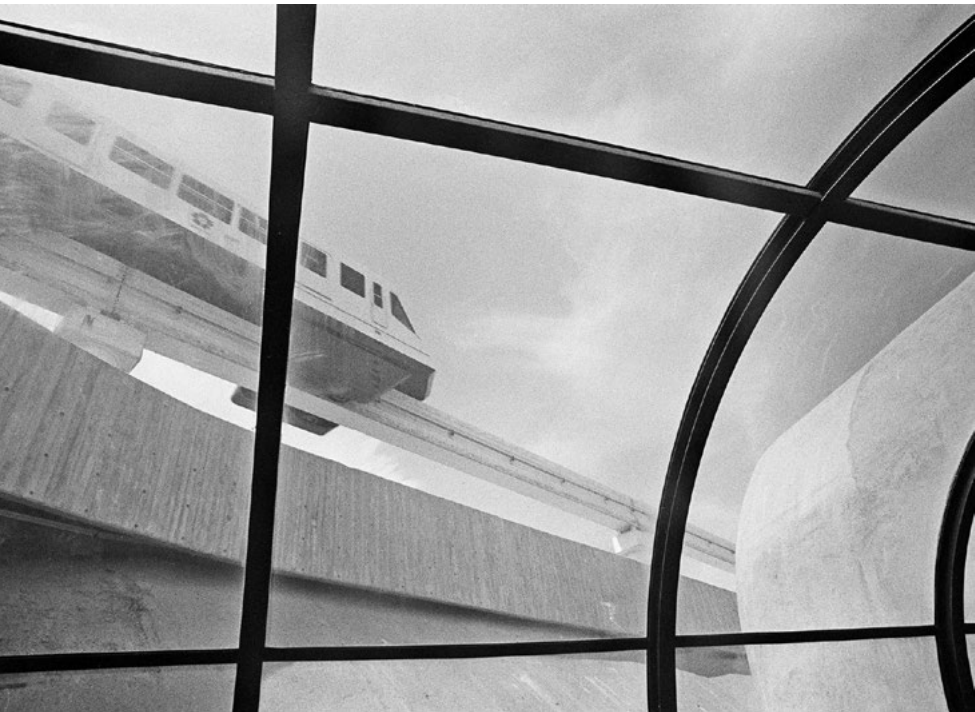
Figure 5.11. Mark Strizic, Monorail Viewed from Inside the Australian Pavilion, Expo '70, Osaka, 1970 .
