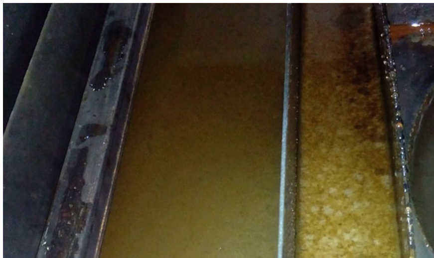
Fig. 5 Petroleum products emergence in the first and the second sections of clarification tank
