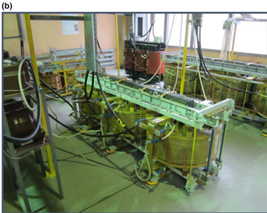
Fig. 1 a Scheme of the physical model and the experimental sample of ACUPF; b Power transformers of physical model and ACUPF; c The phase of the semiconductor switch of ACUPF; d Compartment of ACUPF control system
