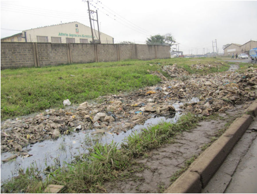
Fig. 18.3 Solid waste blocking drainage systems in Nairobi, Kenya
