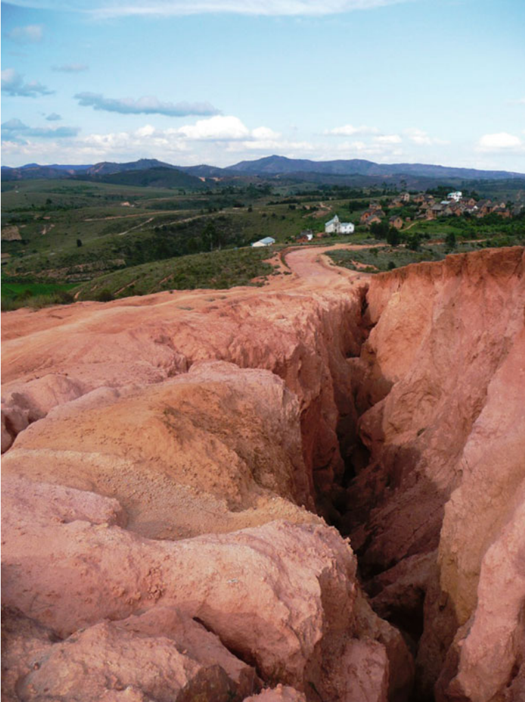
Fig. 7.3 Soil erosion and road degradation in Anjozorobe (north east of Antananarivo)
