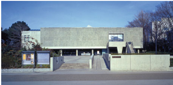
Fig. 14.4 The 4-storey National Western Art (Le Corbusier) Museum in Tokyo, retrofitted by inserting HDRBs in a sub-foundation in 1999. During the 2011 Tohoku earthquake the SI system reduced the PGA values in the two horizontal directions from 0.19 to 0.27 g at the base to 0.08 and 0.10 g at the top (Eisenberg et al. 2011)
