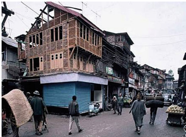
Fig. 1.16 Dhajji Diwari construction in Kashmir, found to have performed much better than more recent forms of construction in Indian Kashmir following the 2005 Kashmir earthquake (Langenbach 2000)
