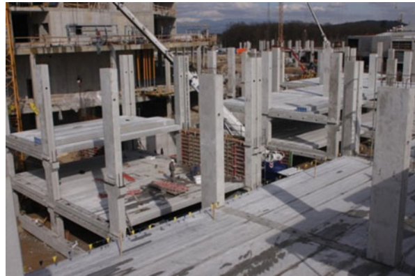
Fig. 4.4 Structural system consists of an assemblage of cantilever columns tied together with beams and floor structures
