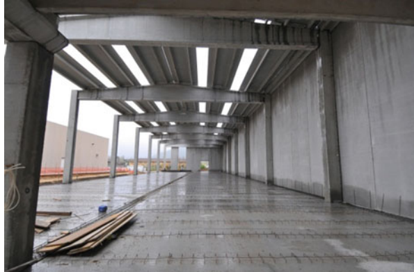
Fig. 4.1 Undamaged structural system of the precast industrial building after the L'Aquila 2009 earthquake
