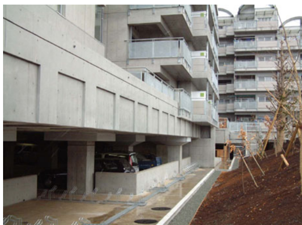
Fig. 14.6 Lateral view of a complex of twenty one 6- to 14-storey buildings, all erected on an unique “artificial ground” isolated at Sagamihara (Tokyo area) with 48 LRBs, 103 SDs and 83 BBs (Martelli and Forni 2010). This was the first Japanese application of “artificial grounds”
