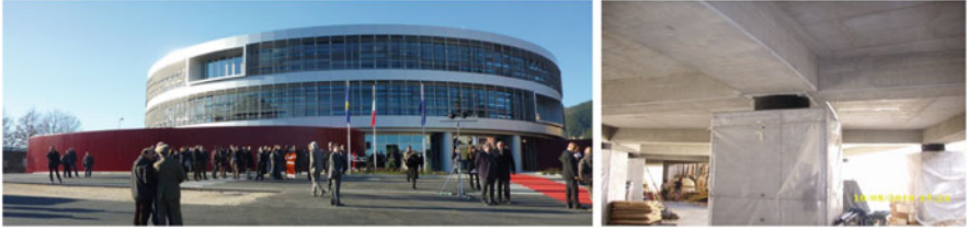
Fig. 14.21 Left : the new Headquarters of ANAS (National Agency for Roads Construction) in L'Aquila, erected on 60 HDRBs after the 2009 Abruzzo earthquake (which had severely damaged the previous headquarters building), completed at the beginning of 2011. Right : view of some of its isolators
