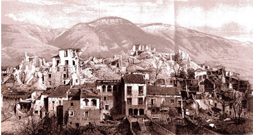
Fig. 1.5 The damage to Polla, in Irpinia, in the 1857 earthquake (from frontispiece of Mallet 1862)
