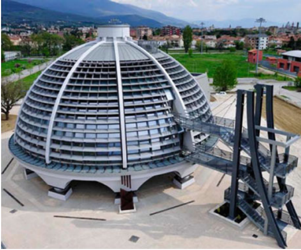
Fig. 14.17 Main building of the Civil Defence Centre of Foligno (Perugia), former seismic zone I, isolated by 10 HDRBs and certified as safe by A. Martelli in 2011
