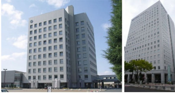
Fig. 14.3 Left : the seismically isolated 10-storey Hachinohe City Hall, near Sendai, isolated by means of LRBs. Right : the 18-storey MT Building in Sendai, isolated by means of RBs and SDs. Both buildings withstood the 2011 Tohoku earthquake undamaged (Eisenberg et al. 2011)
