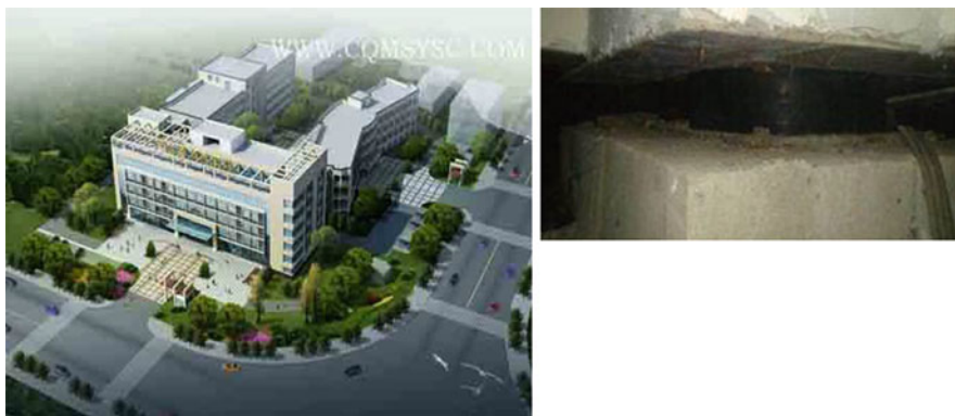
Fig. 14.9 View of the Lushan county hospital (China), before the earthquake of April 20, 2013 (Zhou et al. 2013)
