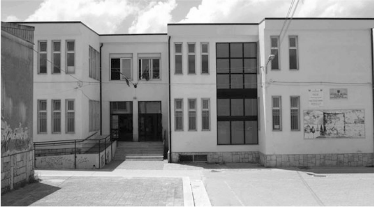
Fig. 3.10 North-east view of the building
