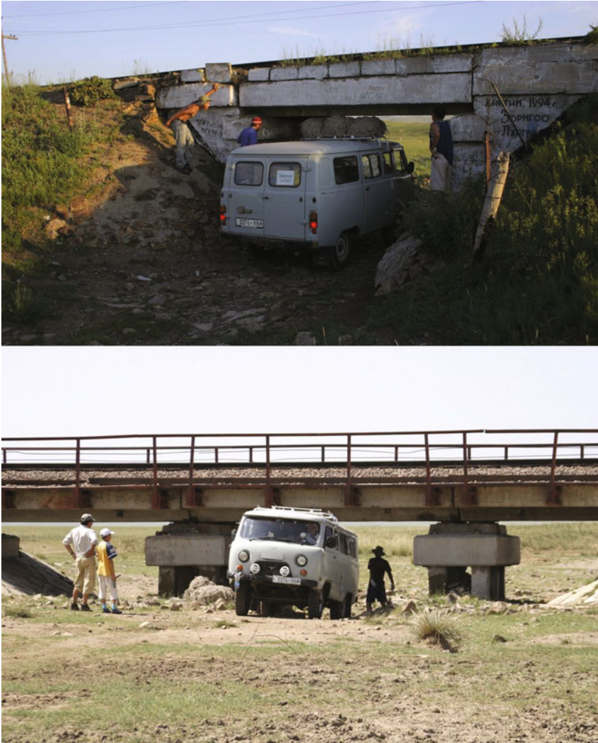
Fig. 14.4 Underpasses on the Ulaanbaatar–Beijing Railway
