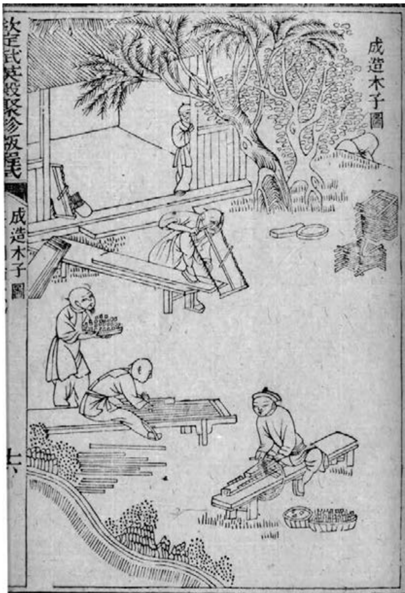
Figure 20 Sawing the wooden types
