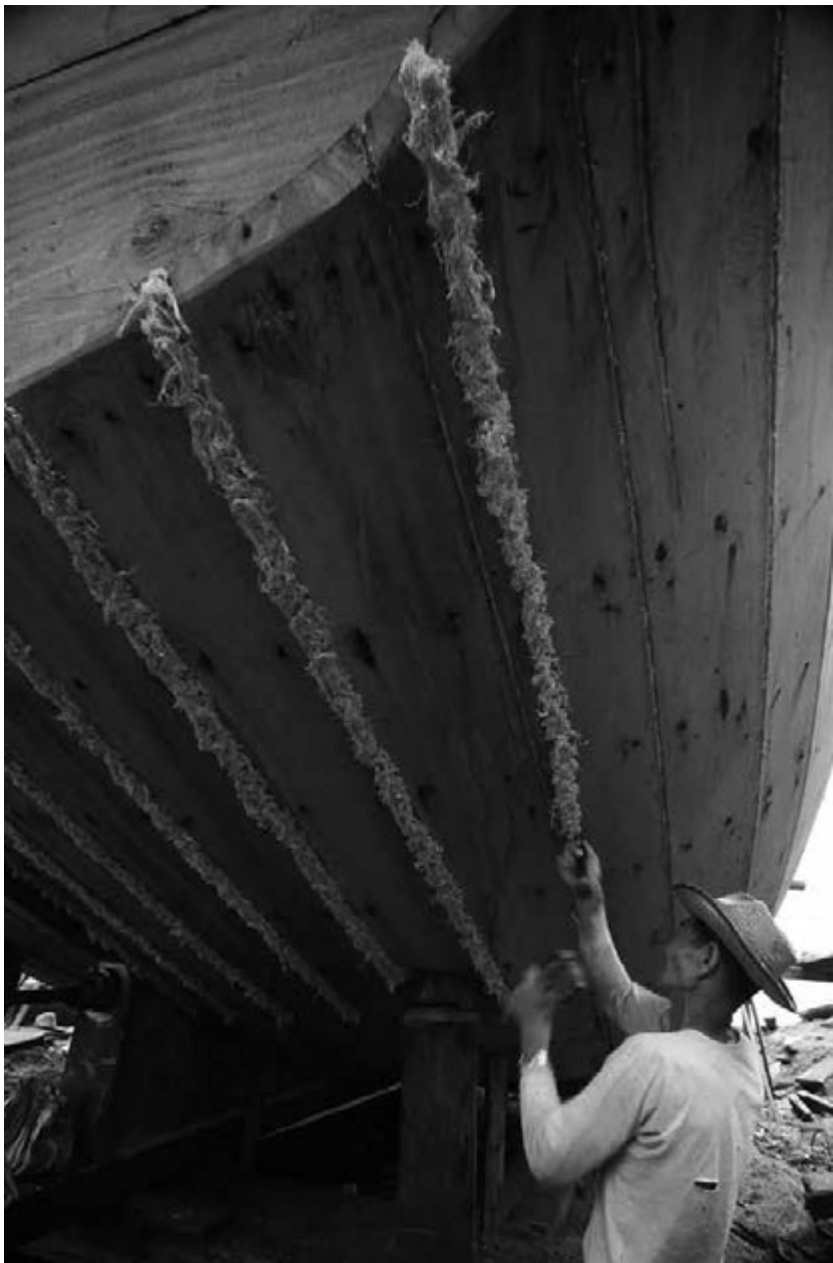
Figure 9 The caulking procedure
