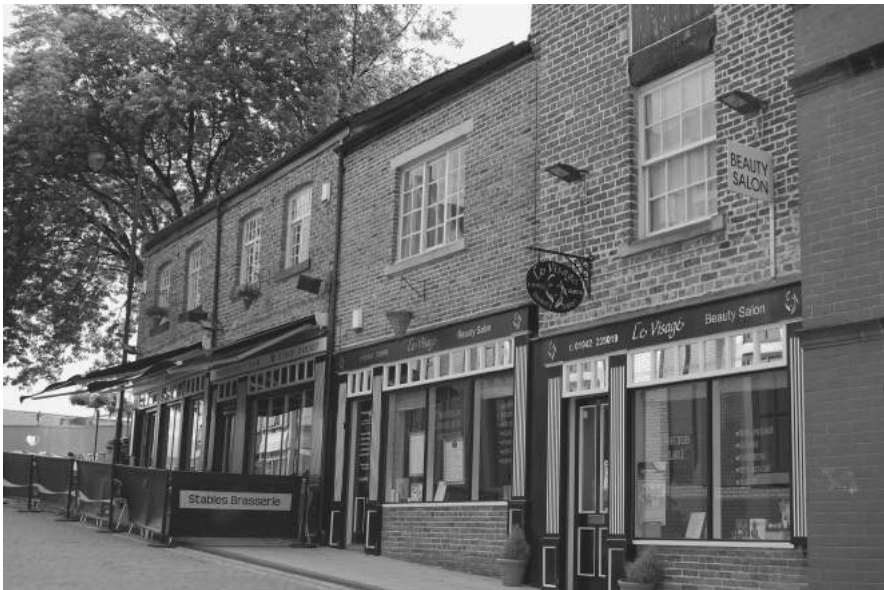
Figure 5.2. Row of shops on Millgate, Wigan, 2010.
