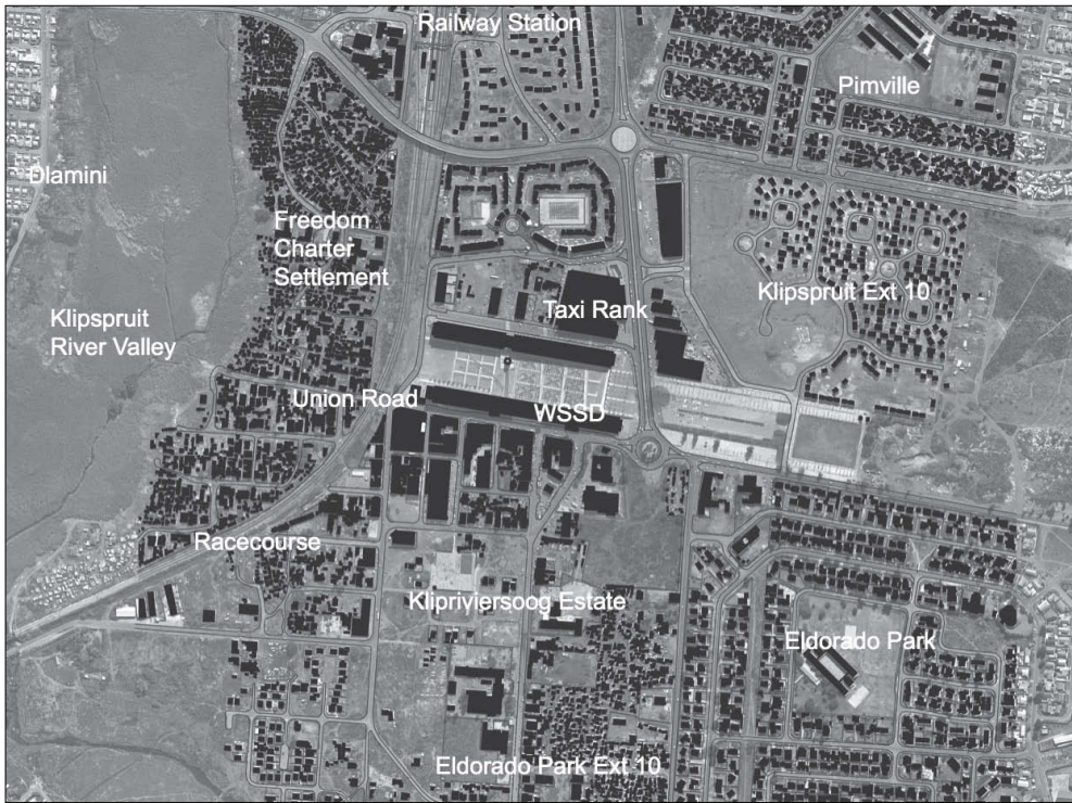
FIGURE 16.1: Kiptown transgresses the definitions of urban or rural, with dense human settlements alongside more open areas, some of which are used for animal husbandry. Its famous Freedom Square, now occupied by the Walter Sisulu Square of Dedication (WSSD), is at the centre of the image. Source: Cohen, Judin and Silverman (2009)
