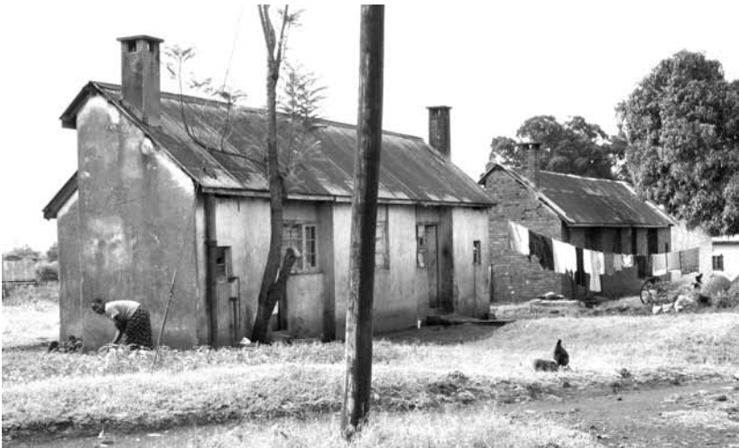
Figure 12.9: Urban Housing Estate in Shauri Moyo Kisumu Where DVBD Staff Lived With Their Families in the 1960s (author's photograph).
