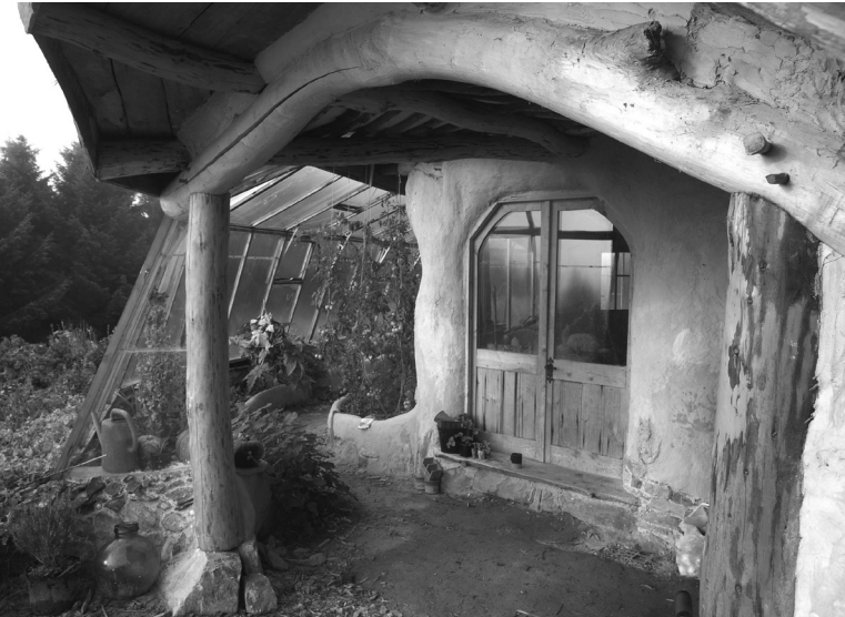
Figure 6.1 Exterior of a Lammas dwelling
